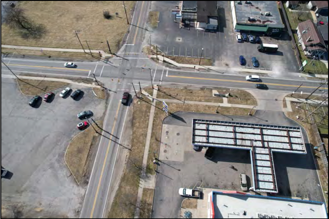
Williams Road, looking west, at the intersection of William Road at Parsons Avenue.
