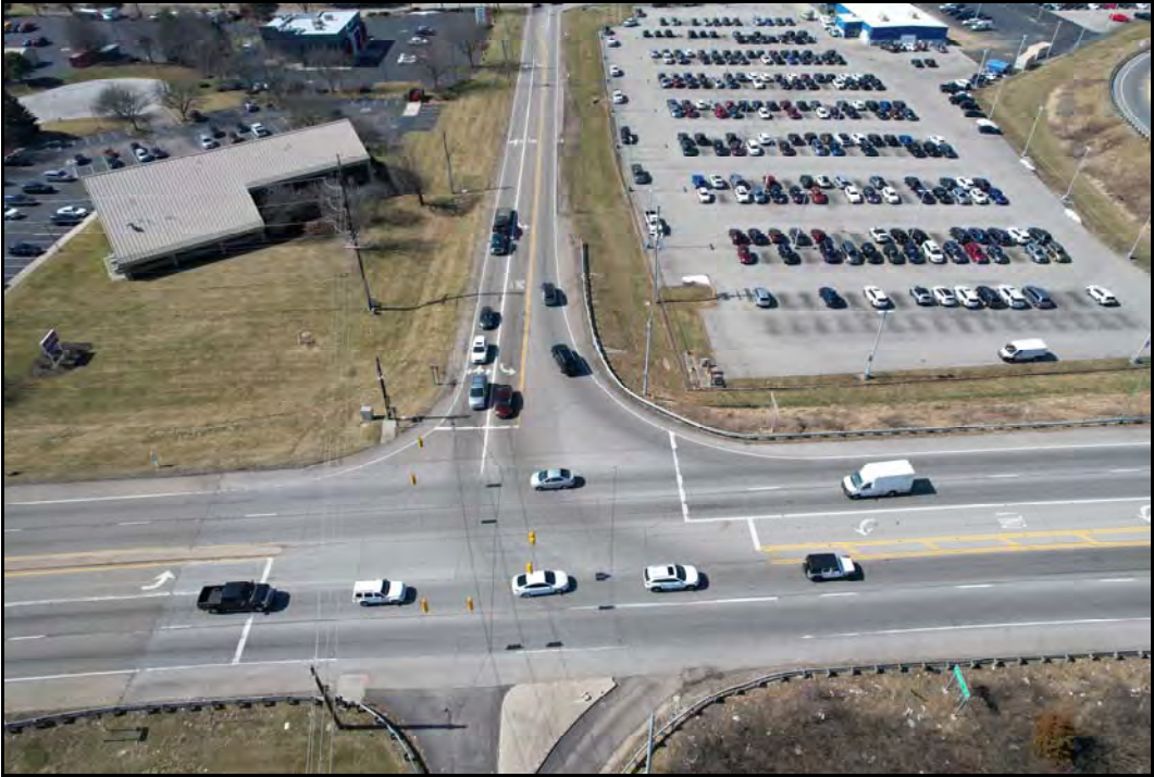
Intersection of Williams Road at SR-317, looking west.
