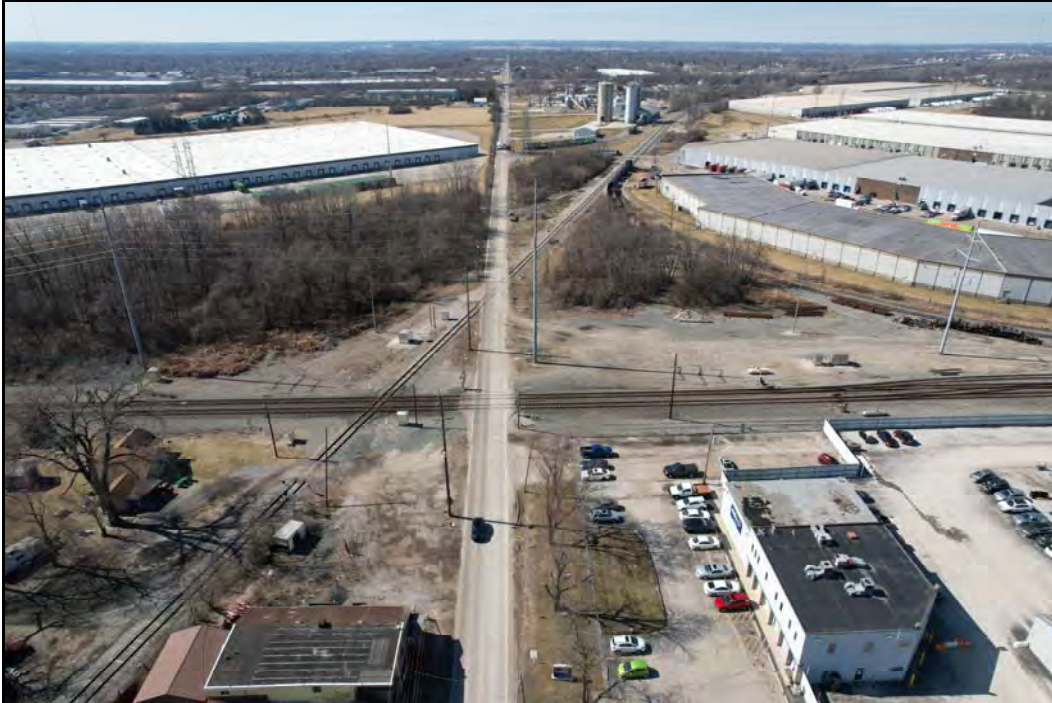
Williams Road, looking west. The two at-grade rail crossings are in the center, with the start of the switching tracks at NS' Watkins Yard's just visible to the north. ODW Logistics is on the north side and XPO Logistics on the south side of Williams Road.
