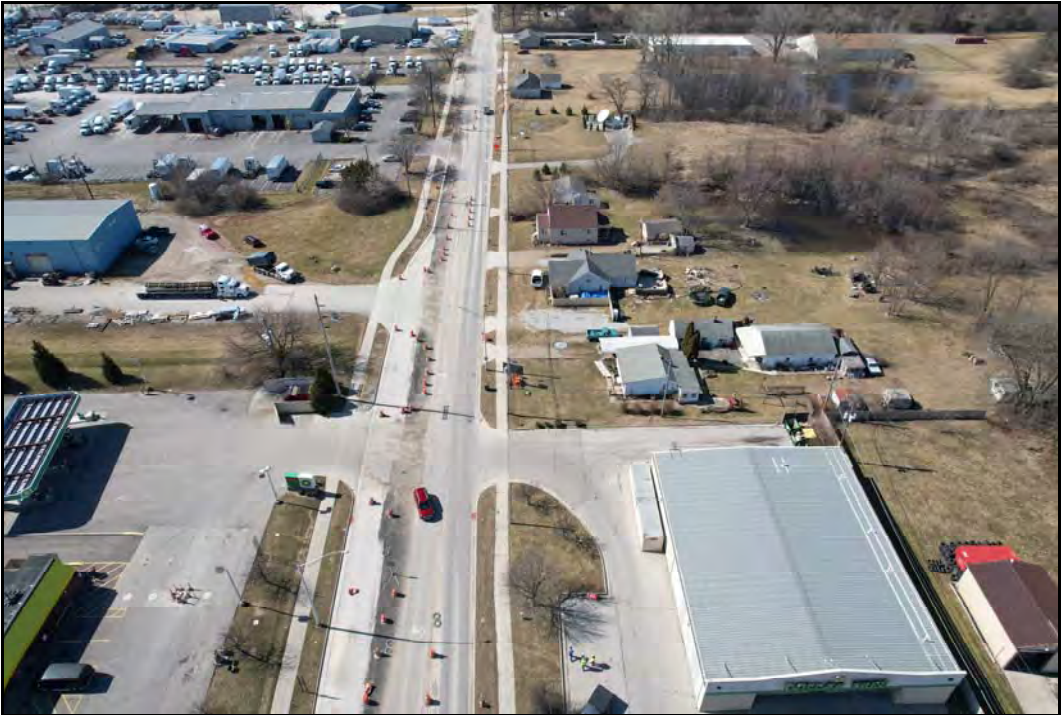
Williams Road, looking west. Residential on north, commercial on south side of Williams Road.
