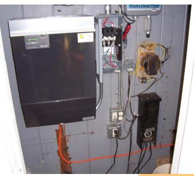
Photos: Brooks Engineering DC Disco is next to inverter, but AC Disco is outside – NO!
