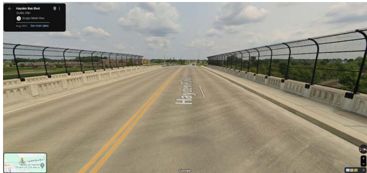
Figure 7-Completed Hayden Run Road bridge over railroad.
