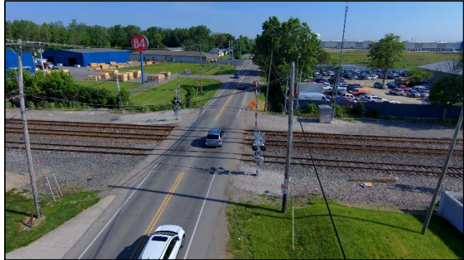
Figure 1-Aerial view of existing at grade crossing (513244C) looking north.
