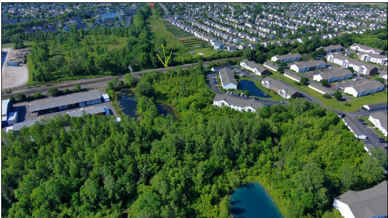
II.2 - Aerial view of looking south towards Galloway Road's current terminus (red arrow), also showing approximate area (yellow arrow) roadway bridge would pass over railroad corridor.
