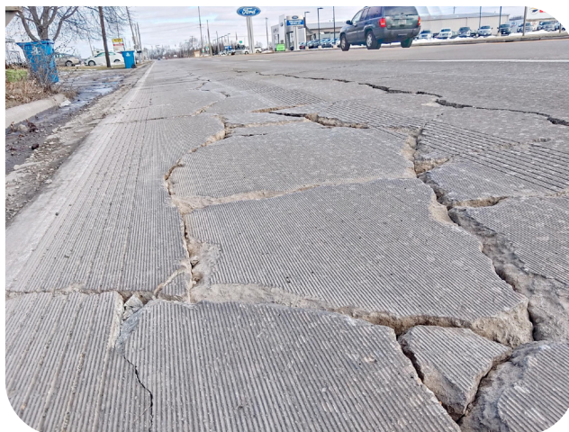
BOTTOM: North Main Street Reconstruction Project
