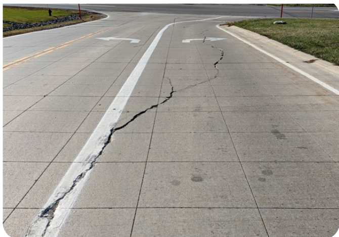
TOP: Christy Road Repaving
