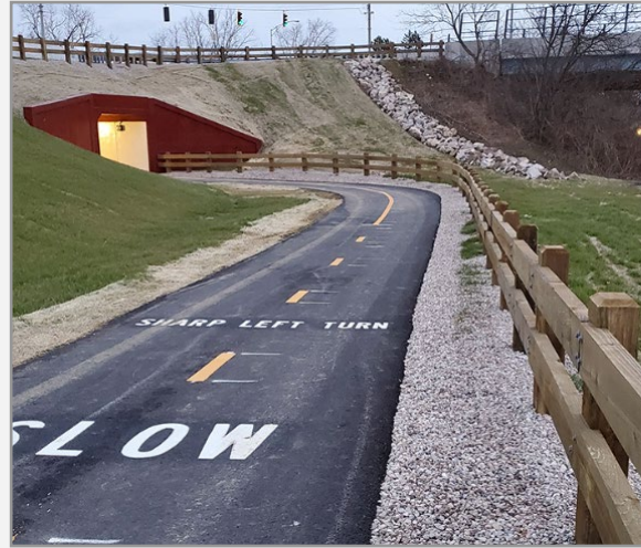
Regional Trail Vision Progress
