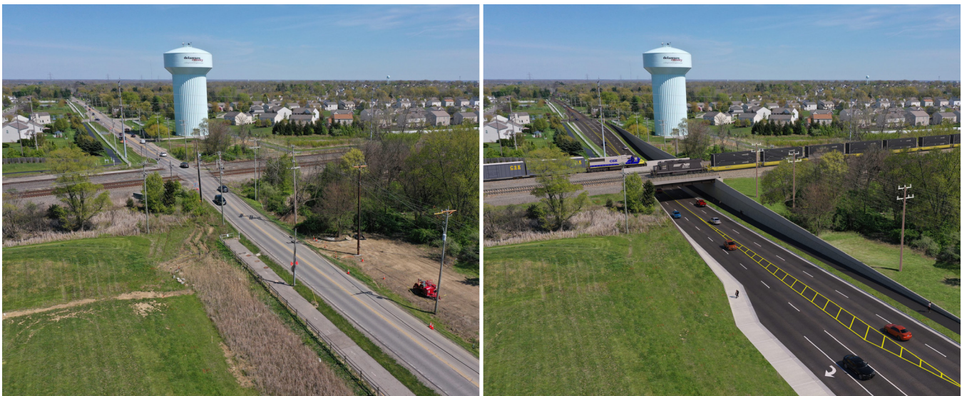
Orange Road today and a rendering of the railroad grade separation. Photo credit: Delaware County Engineer
