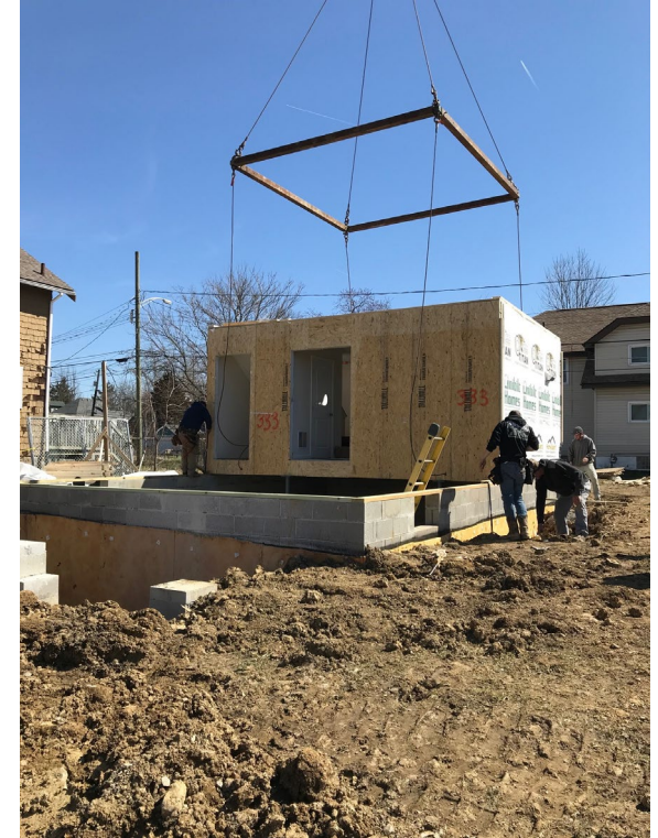
First box being lifted off the semi and onto the foundation
