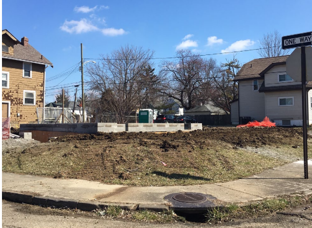
Start of the day, foundation ready...
