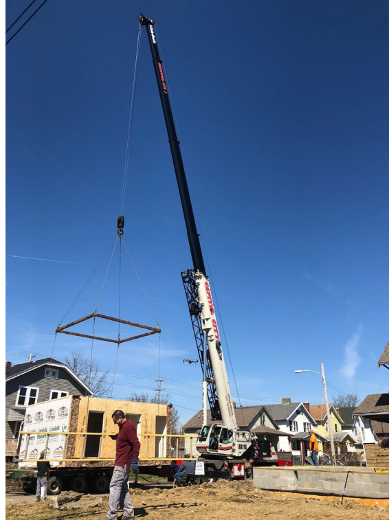
First box being lifted off the semi and onto the foundation
