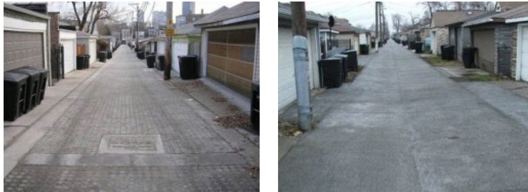
Green Alleys in Chicago (Source: Abby Hall, US EPA)
